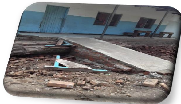
Photo; Construction of Stair Ramp at Kisawasawa Pre-Primary School
