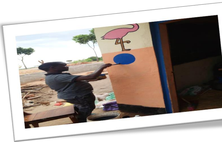
Photo:Ongoing Renovation in Mkindo- B Pre-Primary School
