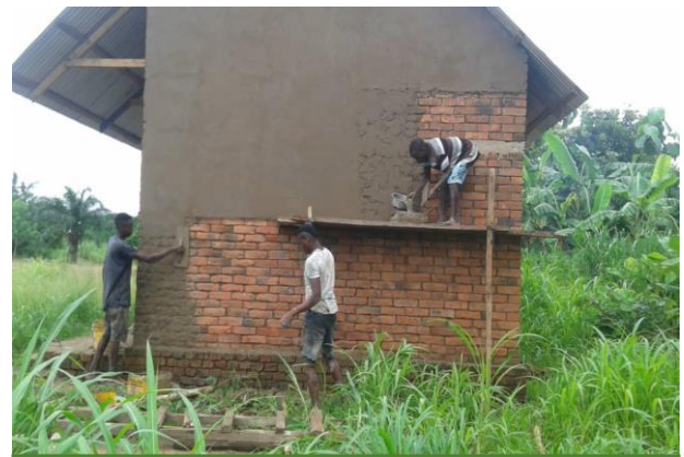
The supported building at Bwawa la Chumvi
